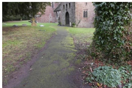
Uneven path from Lych Gate to North Porch
