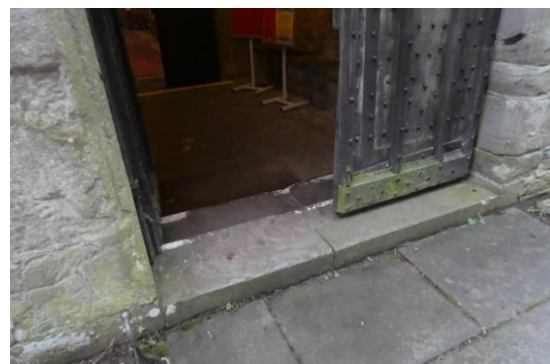
Outer double doors, with a raised threshold with one step up and two steps down inside
