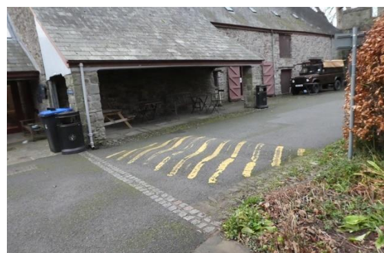
Narrow smooth strip on far side of speed bump in the Cathedral Close is too narrow for easy wheelchair circulation
