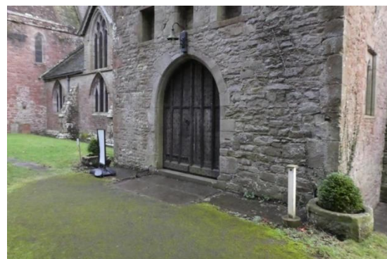
Approach to North Porch and 125mm step at double doors
