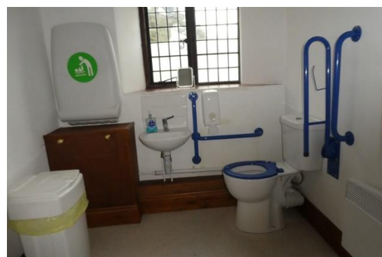
Interior of unisex wheelchair accessible WC cubicle
