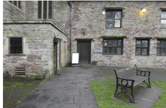
Flagstone path to accessible door into vestry range
