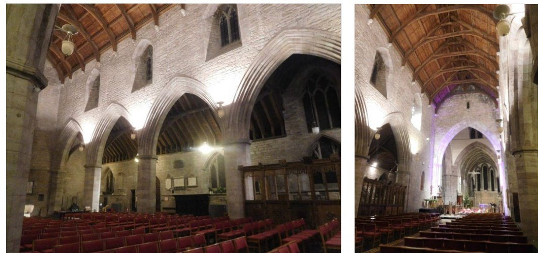
Figure 4: Survey photos of Brecon Cathedral
